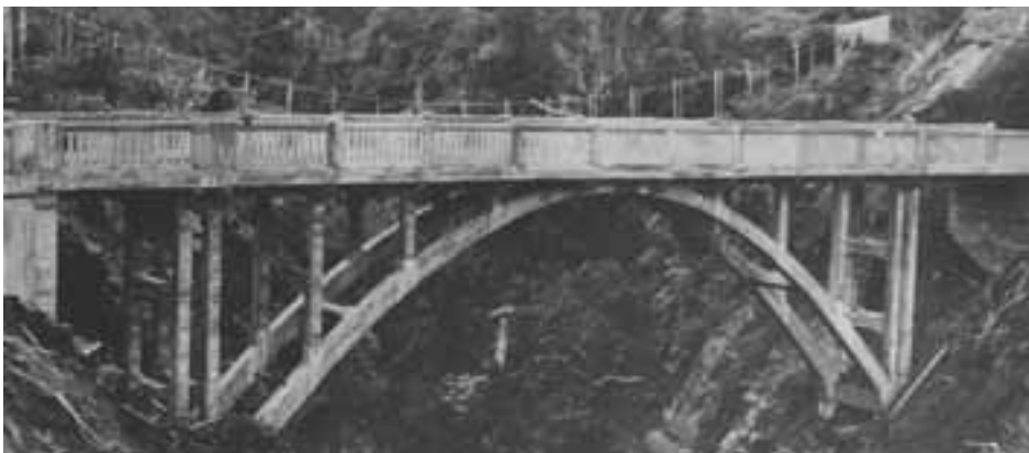
The famous Bridge to Nowhere under construction.
